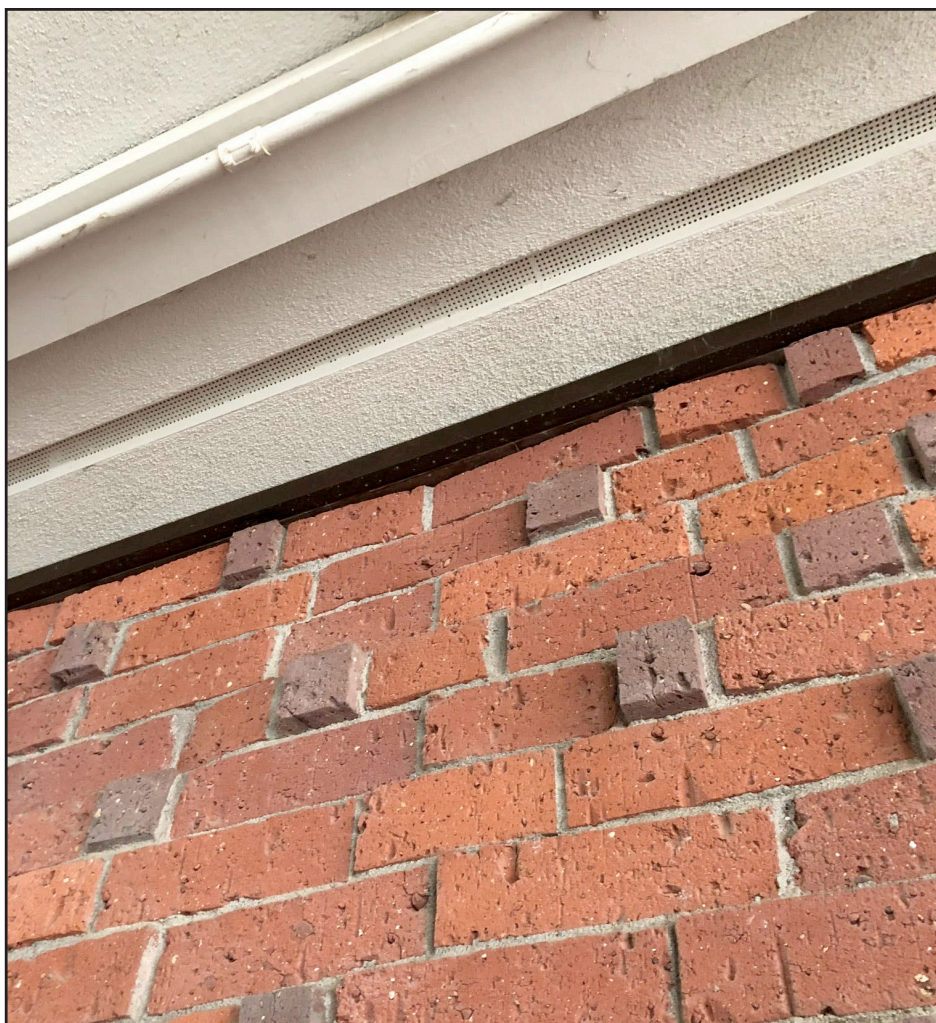
Newly added sealant and edging (along the top of the bricks) helps to close gaps in Kennedy's outside walls. This and other measures are helping to prevent bugs and rodents from getting in. Clarion staff photo
