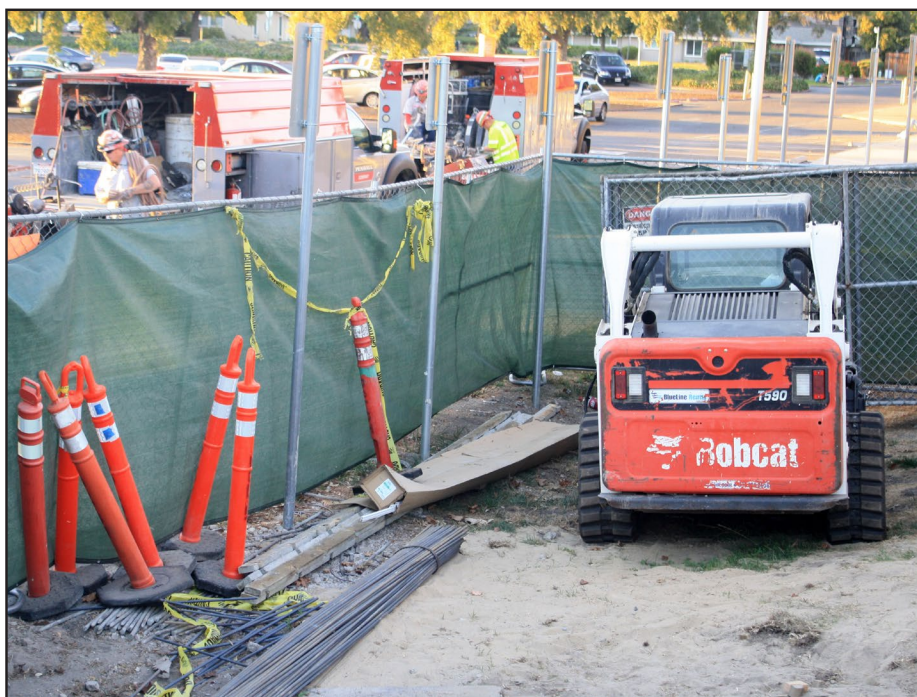
Repair work continues through the month of October on the Kennedy campus. Photo by Joe Temblador, Editor in Chief
